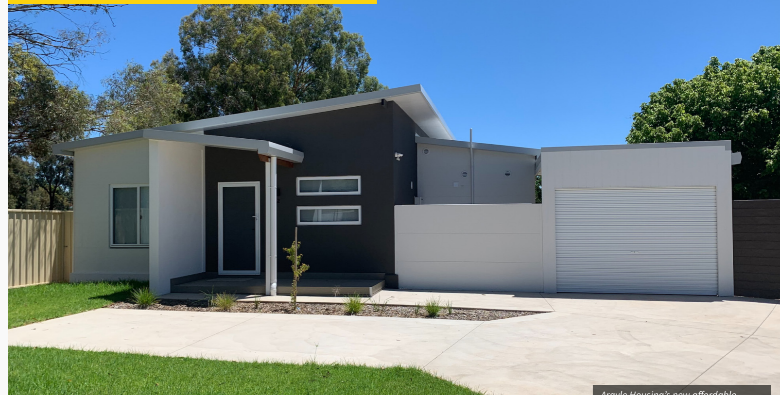
Argyle Housing’s new affordable modular homes in Wagga Wagga NSW
